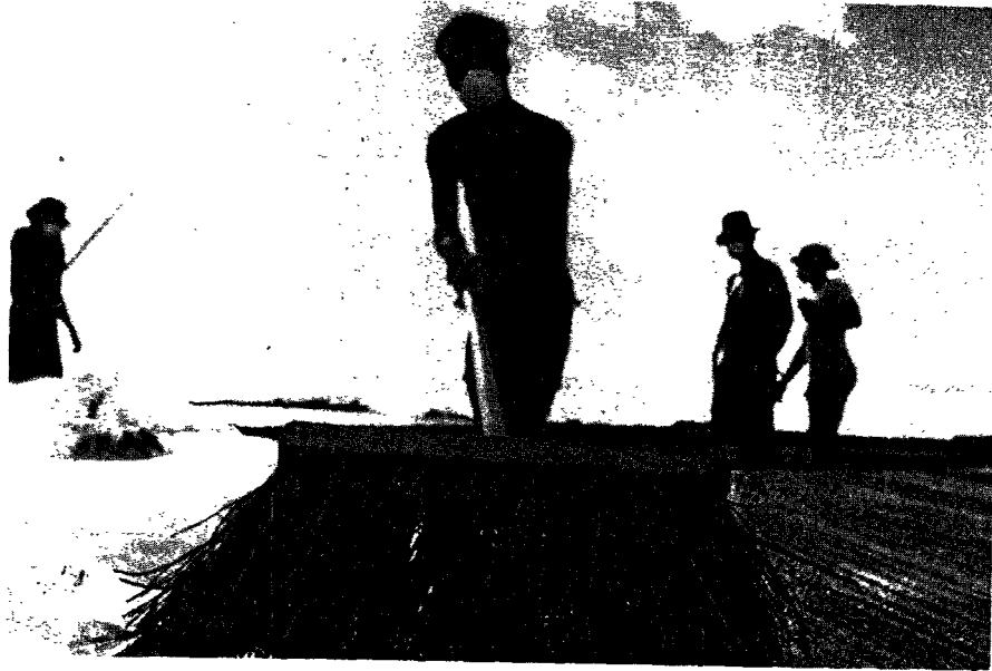
FIGURE 8-48. BROOM-FINISHING A CAP SECTION.
