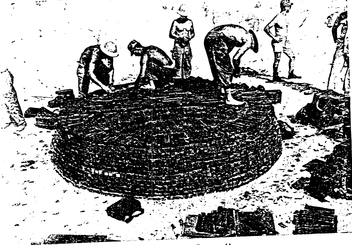
Preparing For a TNT Charge in Program 11
