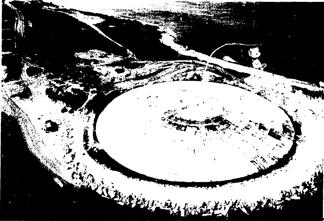
FIGURE 6 The containment structure at time of completion. (Photo courtesy of Defense Nuclear Agency.)
