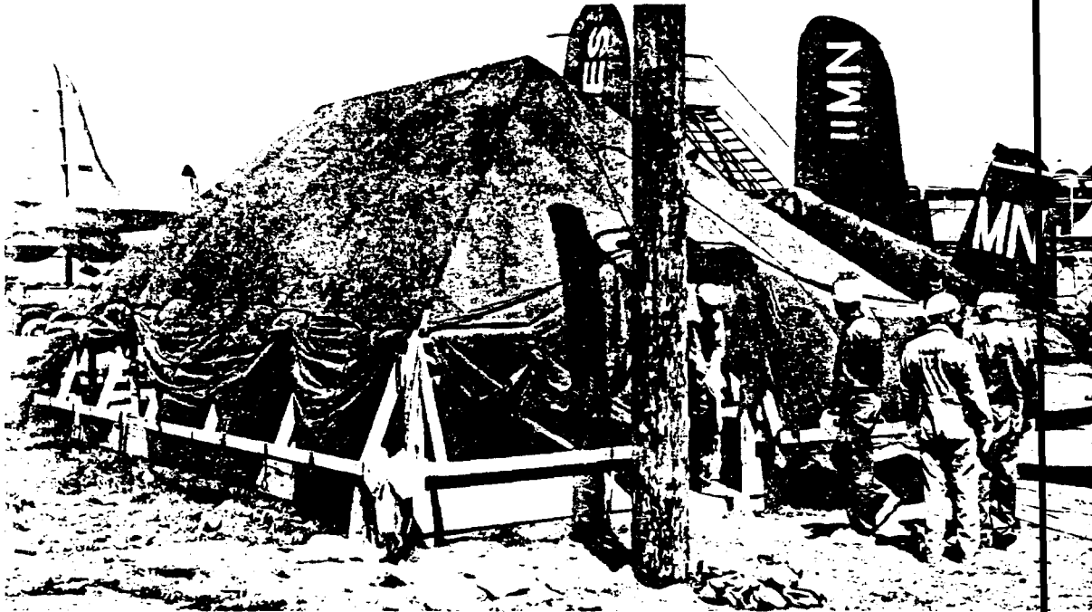
Figure 40. Tent for changing contaminated clothing at Parry, CASTLE aircraft and four unmanned F4U aircraft used in Project 6.4 (Proof Testing of Atomic Weapons Ship Countermeasures) also required decontamination.
