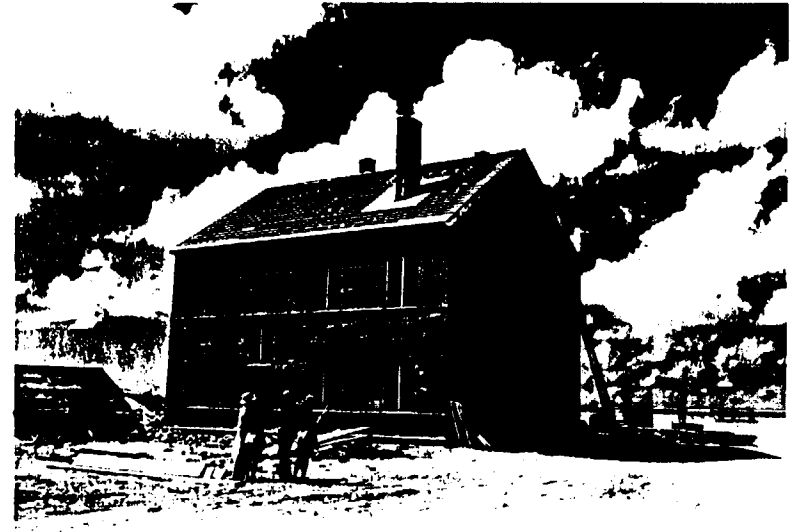
FIGURE 1-47. STRUCTURE-TEST BRICK HOUSE, ENJEBI.
