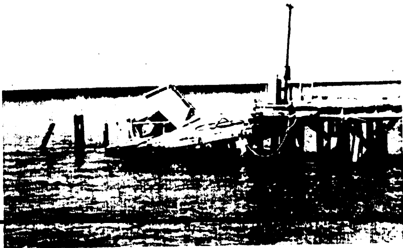
FIGURE 3-2. DELAPIDATED BOAT DOCK.
