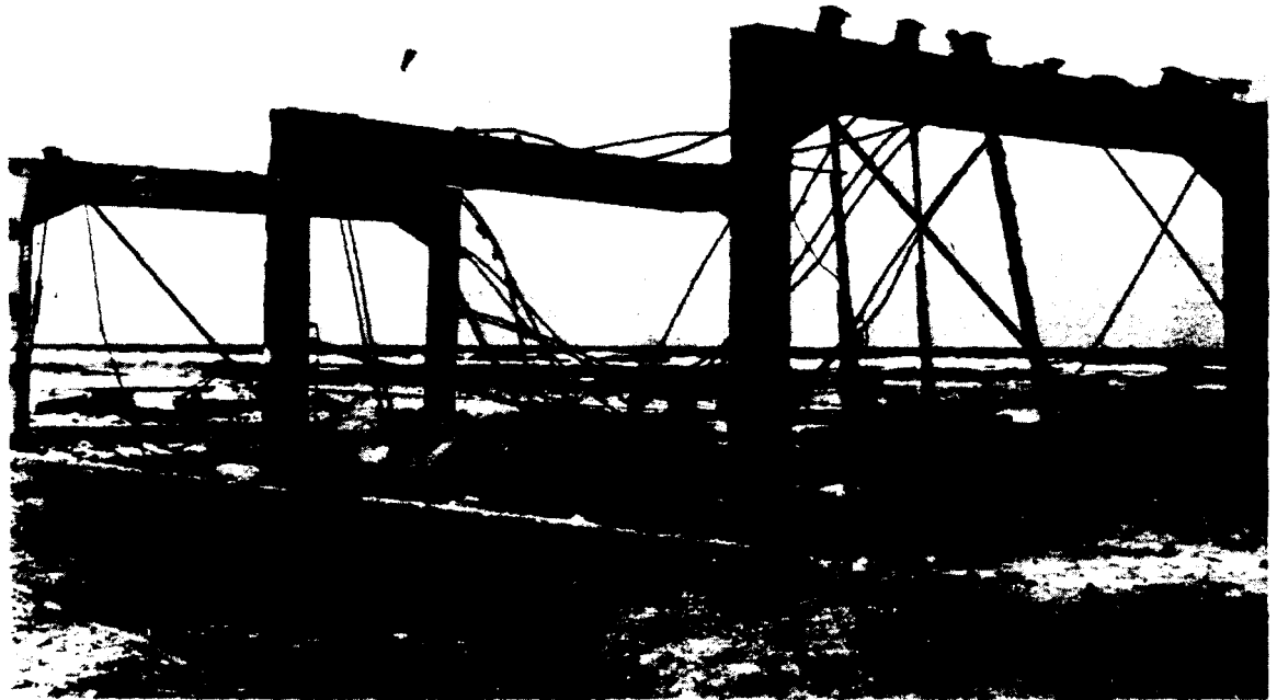
Job 5 Support & Roll-up Program Incuded Disposal of Damaged Structures Such as This Station 3.3.8.
