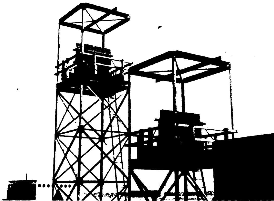
Ganex Towers, Station Nos. 145 & 146, Erected in Front of Station No. 144a.
