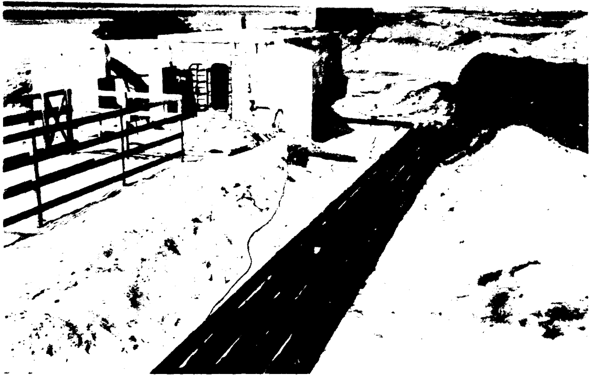
Six-Inch Conduit Installation Between Scientific Station 69 & 6b, Biijiri
