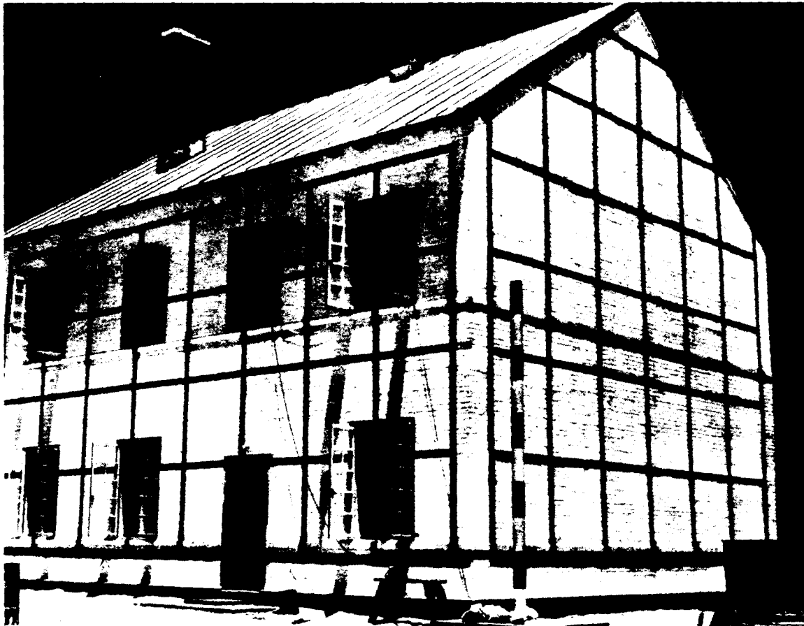
Front Elevation of Brick House, Military Structures Program, Station 3.3.5a (Air Force) on Engebi.
