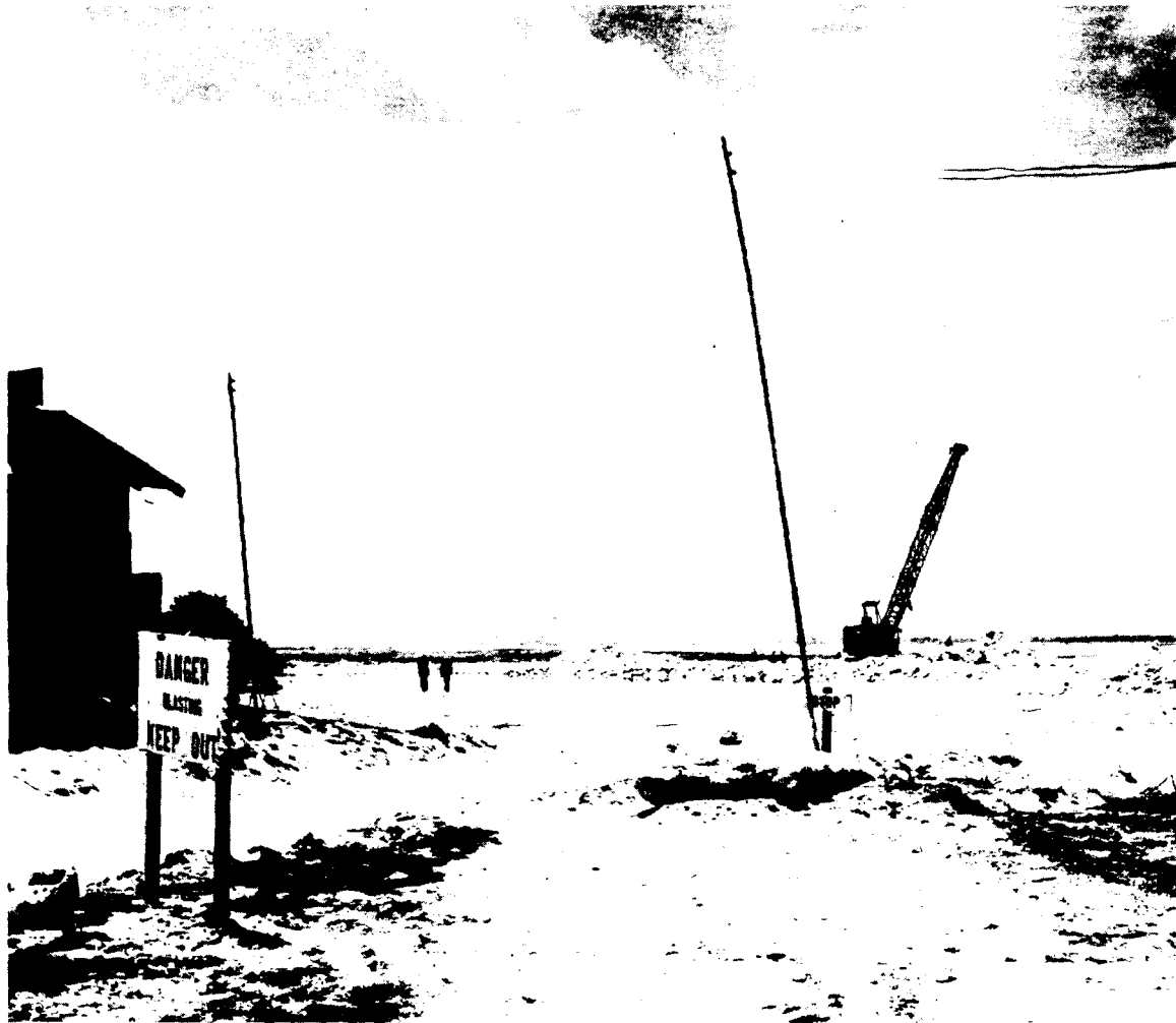
Blasting Coral Ledge on Reef to Obtain Rock for Crusher Plant.
