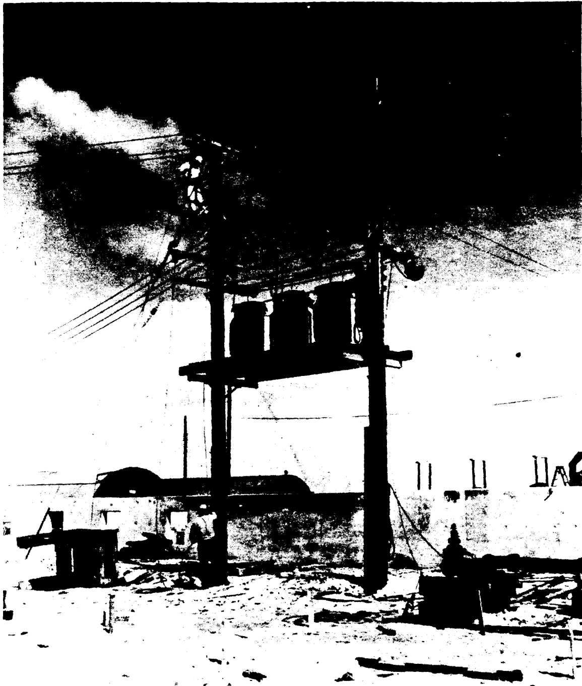
Connecting Transformer Bank for Overhead Power Distribution System, Parry Island.
