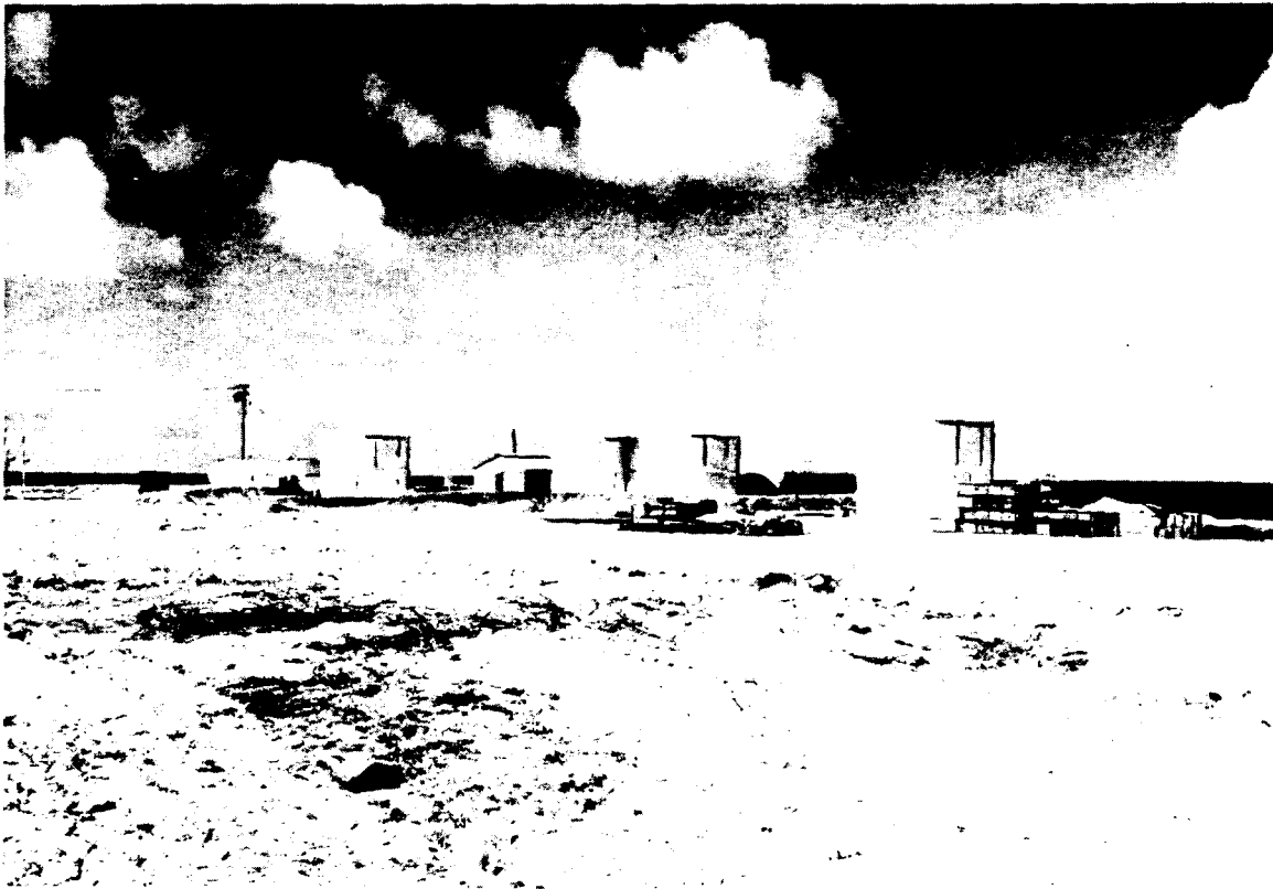
POL Tank Farm, Parry Island, Showing Part of Tanks Installed, Pump House in Background.
