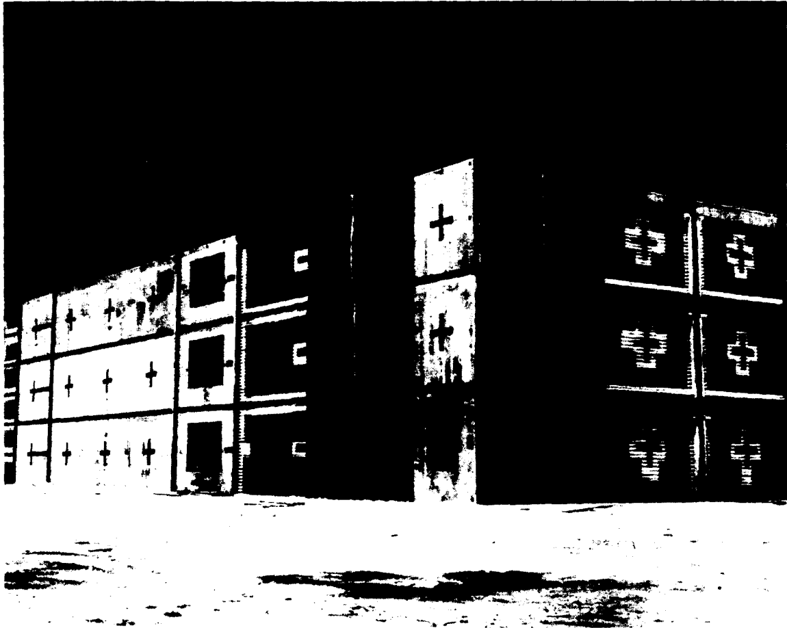
Engebi: Military Structures Program, Station 3.1.1 (Army), Front View of Completed Building.
