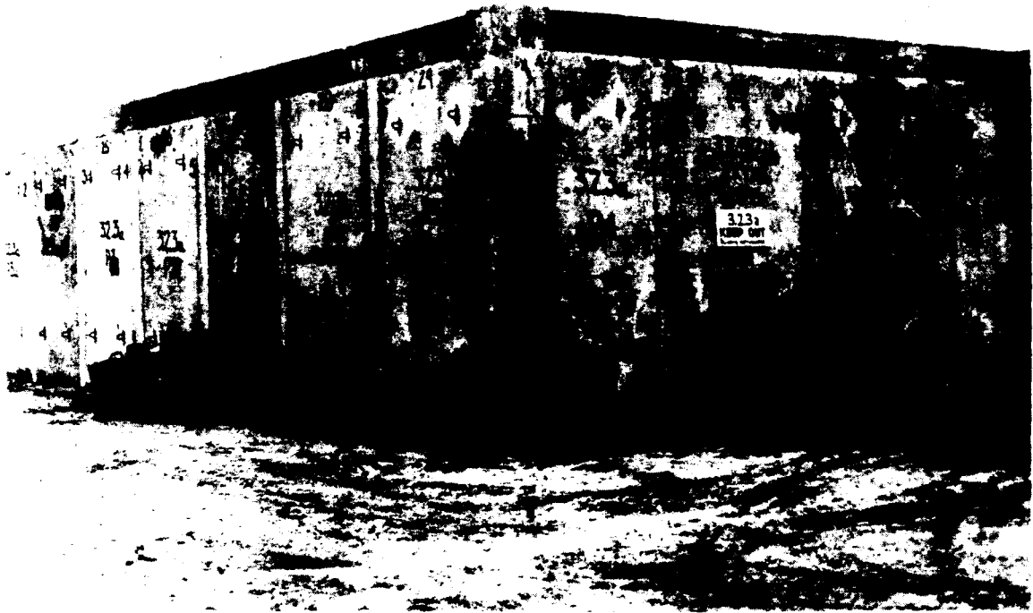
Military Structures Program, Station 3.2.3a (Navy). Precast Concrete Sections.
