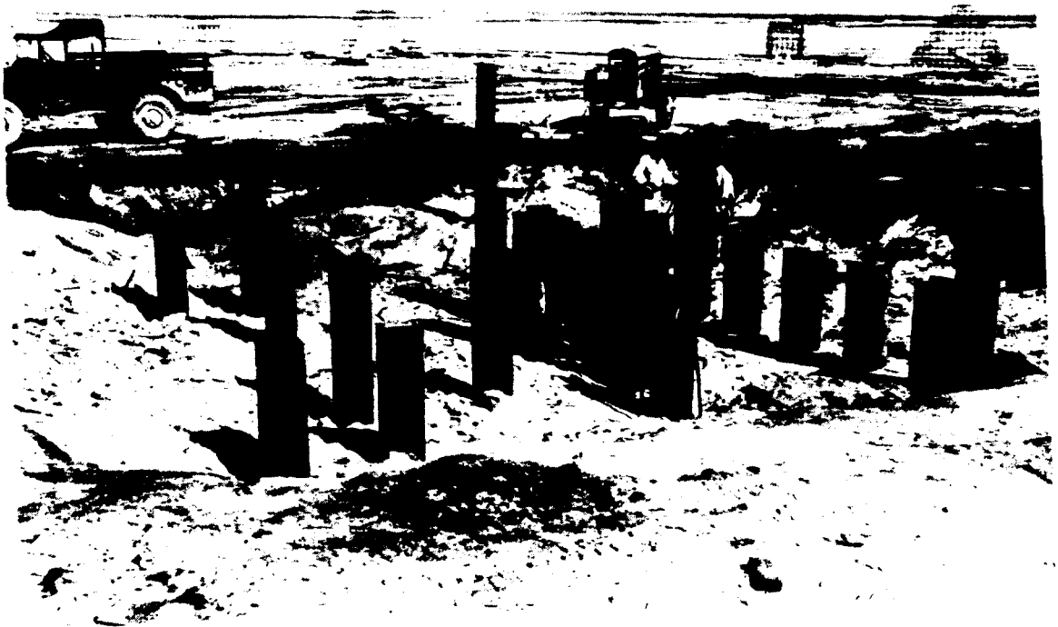
H-Beam Piling in Place for 200-ft. Tower on Ebiriru.
