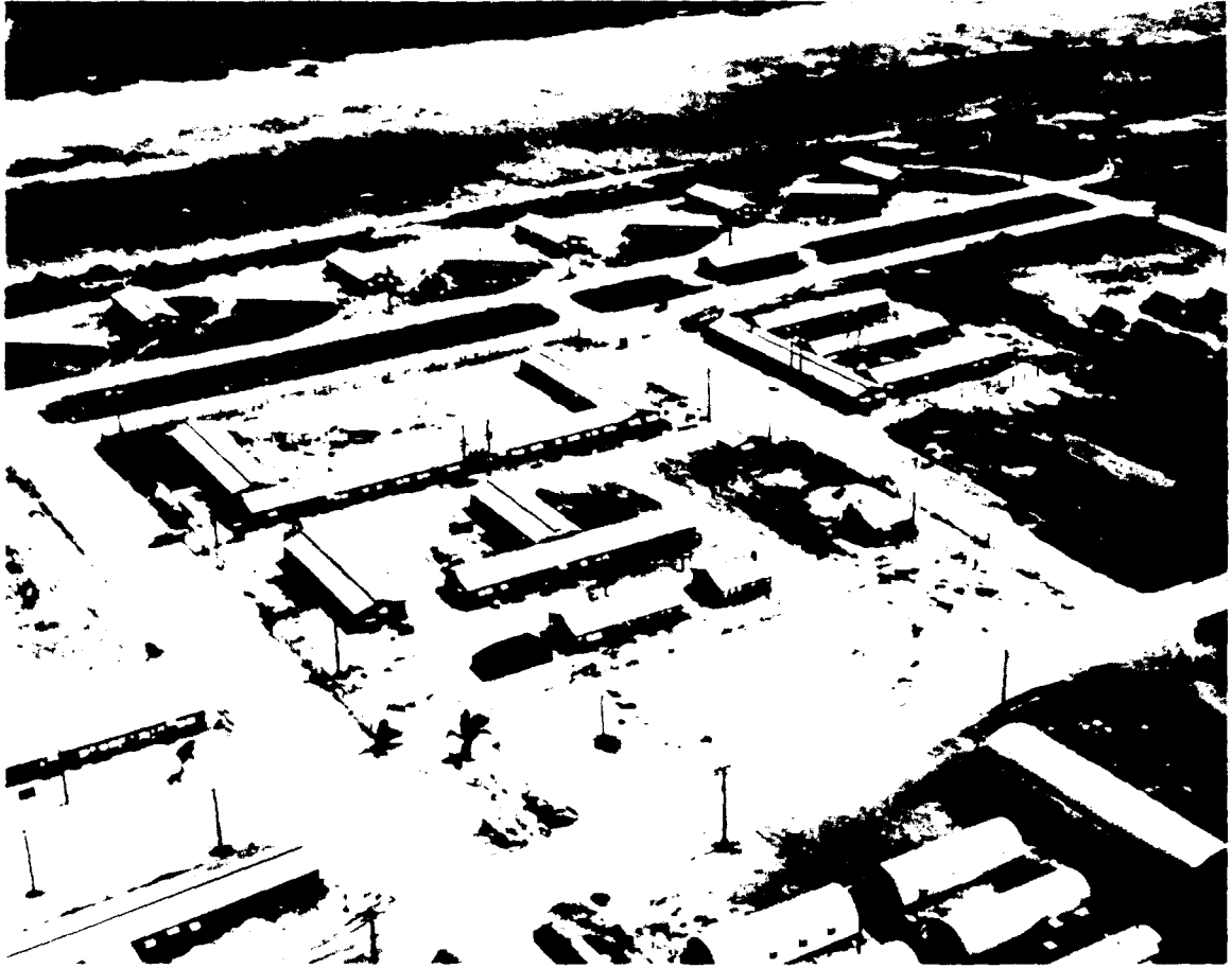
Aerial View, Parry Island, Showing Quonsets, Administrative Area Security Compound, and Personnel Barracks
