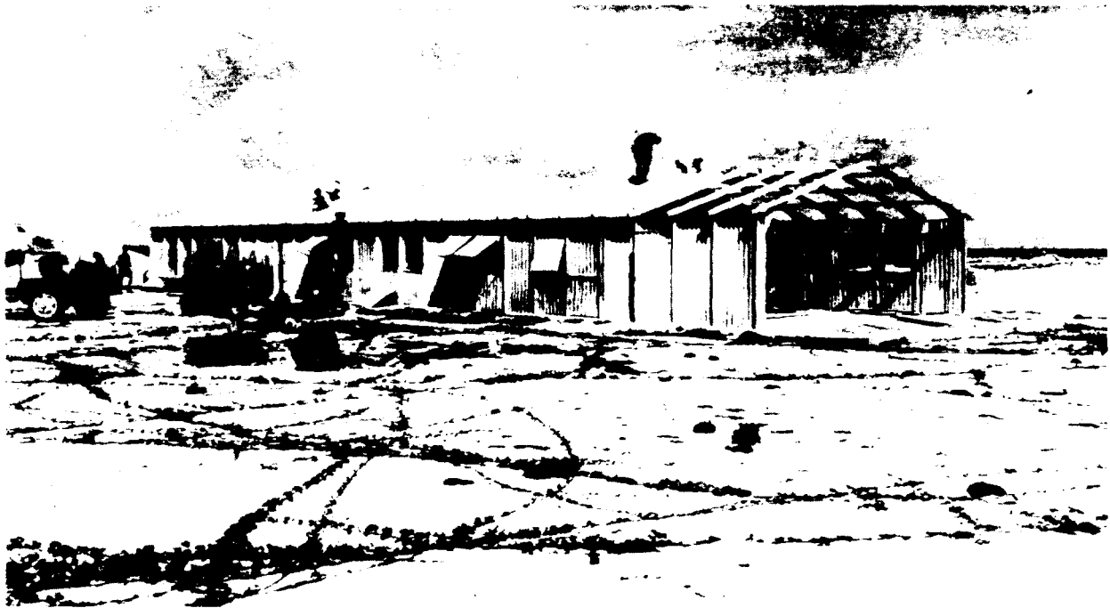
Figure 2-33. Yvonne Mess Hall Under Construction
