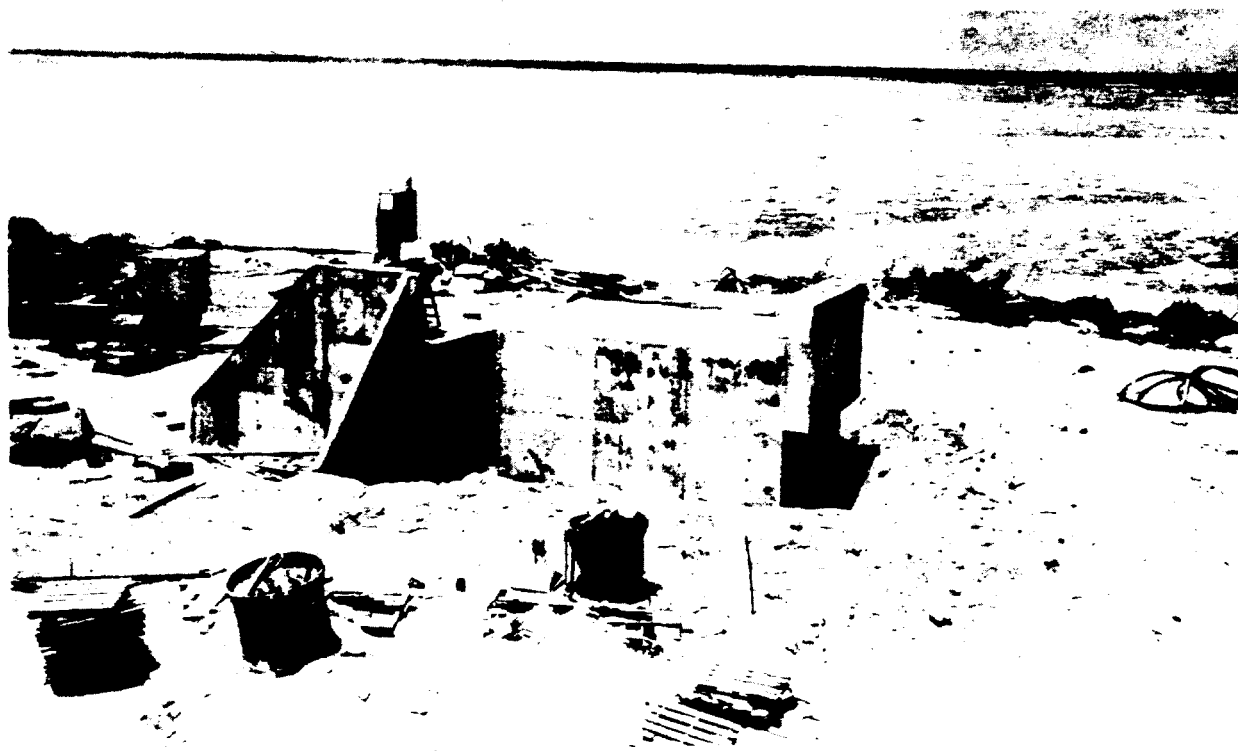
Figure 2-86. Entrance Side of Station 520 During Construction
