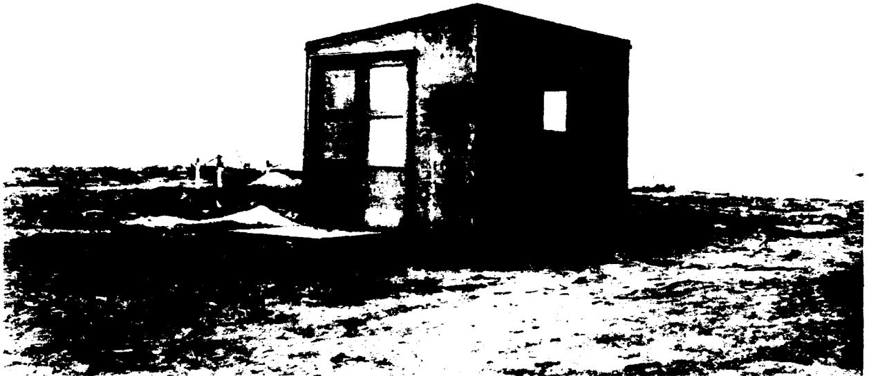
Figure 2-77. Station 3 During Construction
