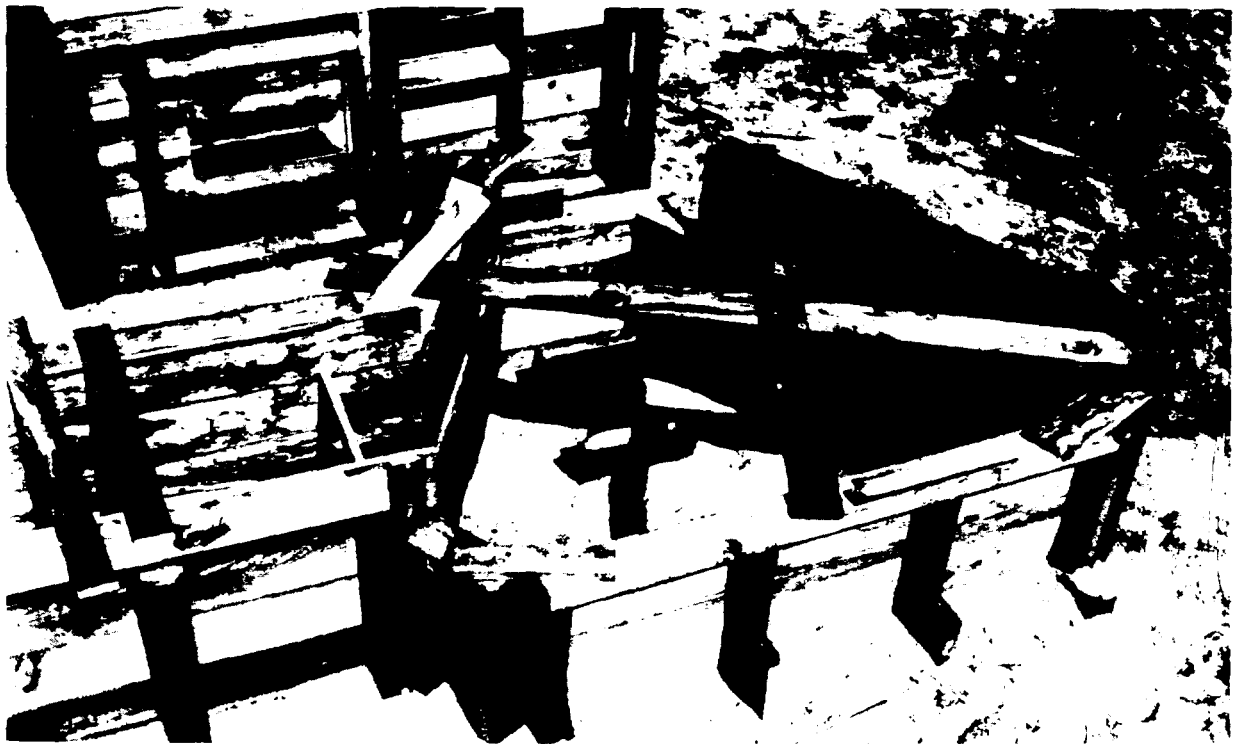
Figure 2-70. Pile Pad Form, Station 1
