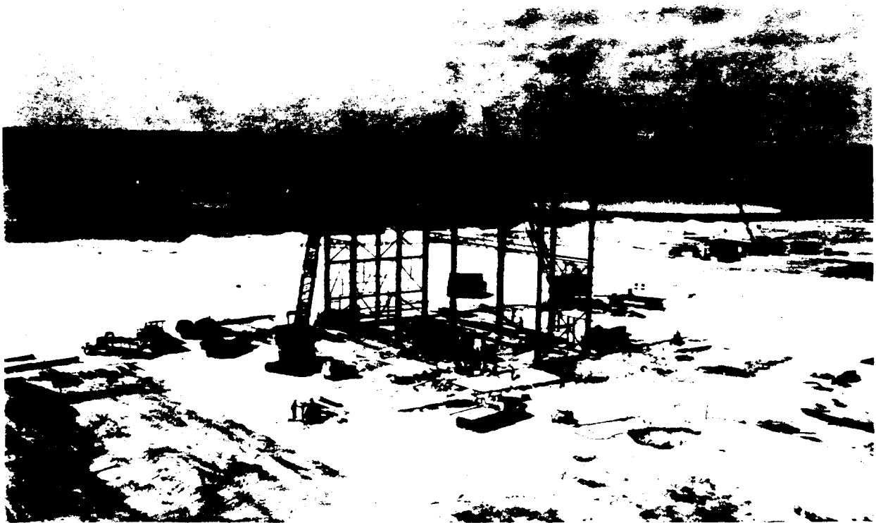
Figure 2-72. Erection of Columns for Station 1
