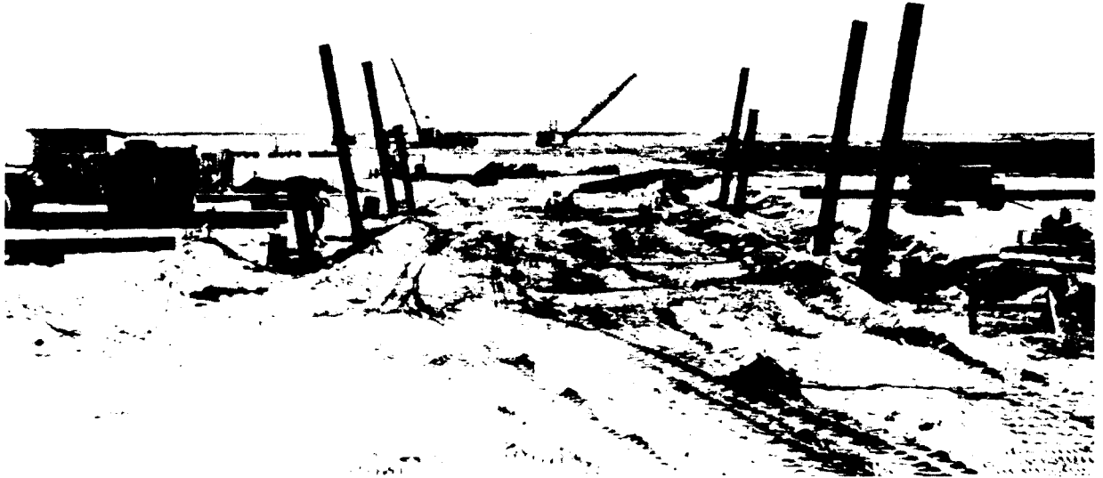
Figure 2-69. Batter Piles Driven 60 Feet Deep, Station 1
