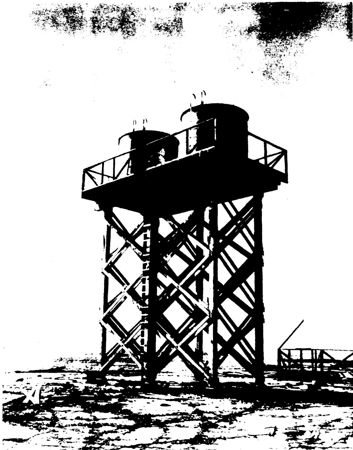
Figure 2-37. Water Tower Re-erected at Yvonne
