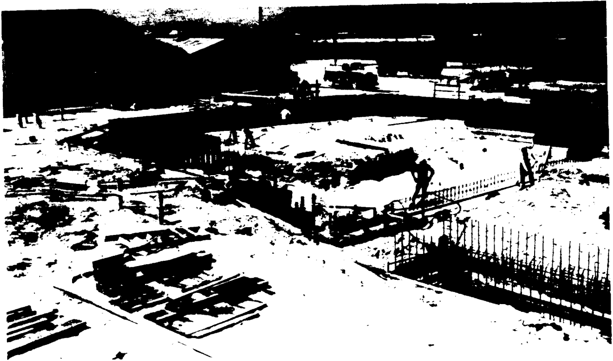
Figure 2-47. Placing Reinforcing Steel for Bldg. 344
