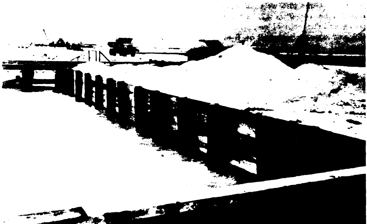
Figure 2-32. Jetty Bulkhead and Fill at Gene
