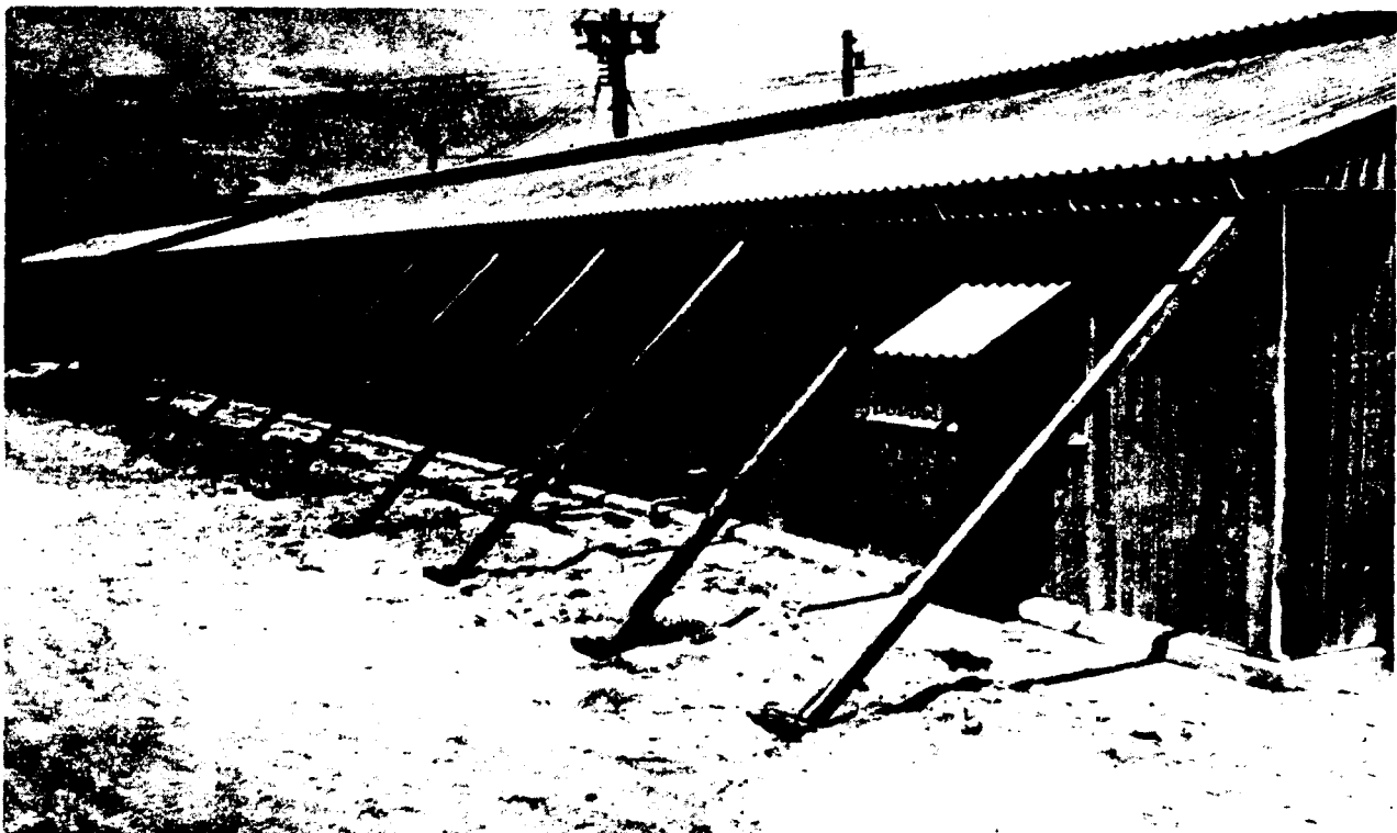
Figure 6-4. Typical Exterior Building Bracing
