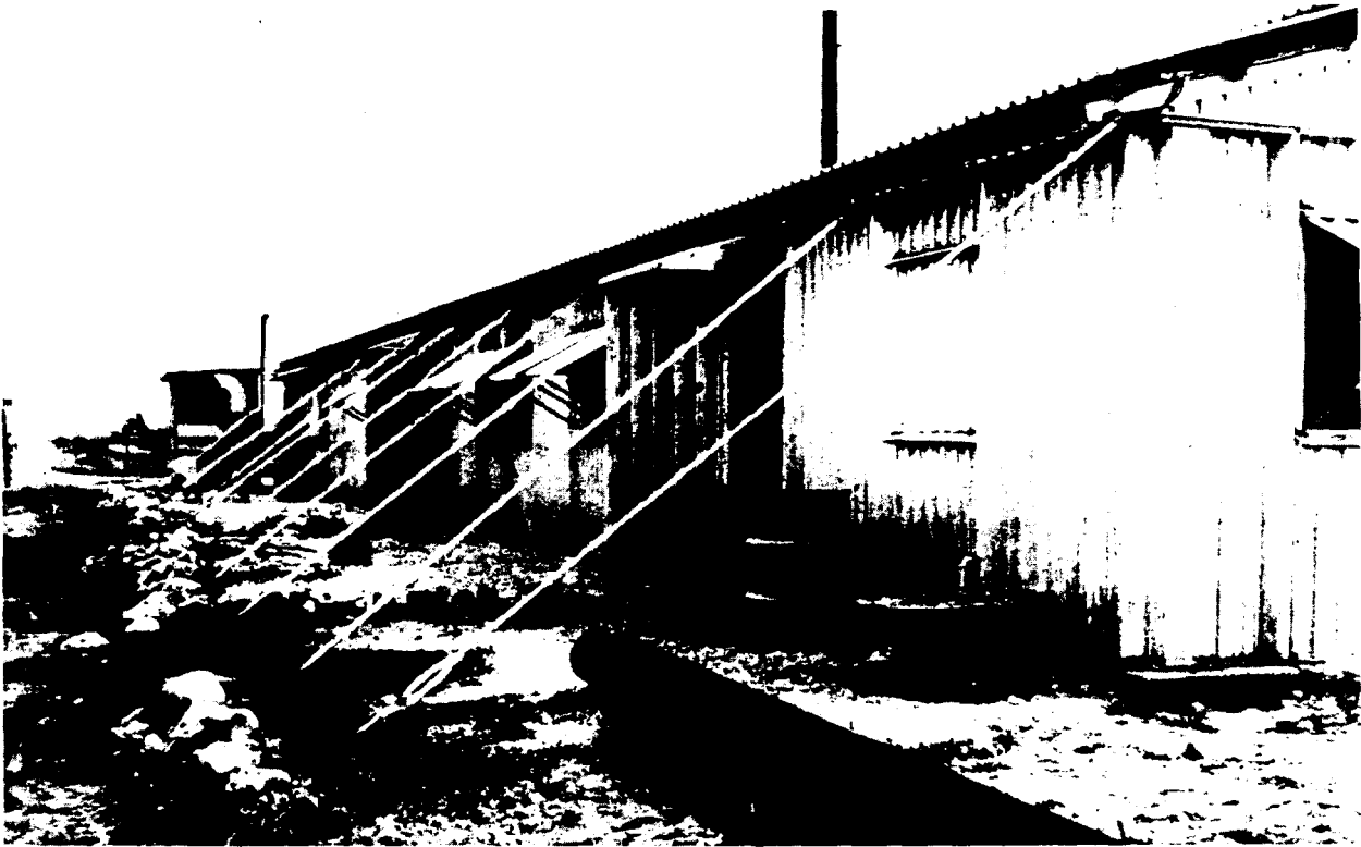
Figure 6-2. Guy Bracing on Exterior of Building
