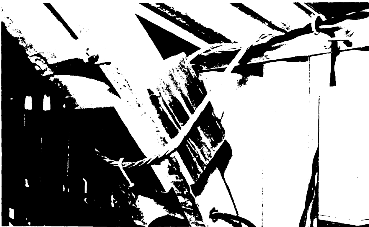
Figure 6-3. Typical Guy Anchorage in Building
