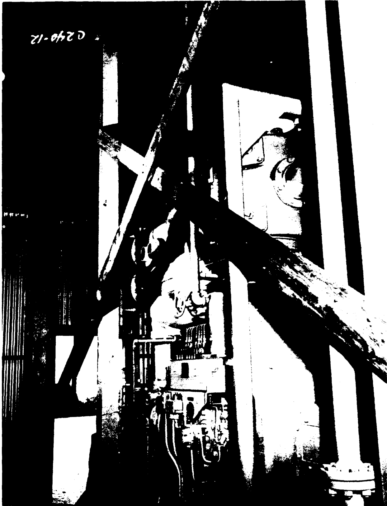
Figure 6-8. X-Bracing to Roof Support in Cryogenics Building
