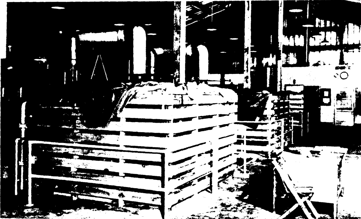
Figure 6-11. Cribbing Around Power House Generators, Elmer
