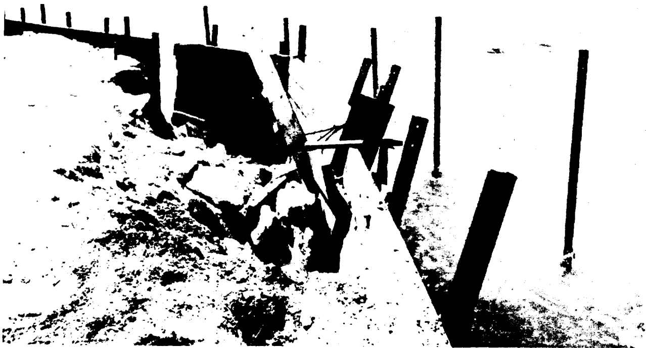
Figure 2-214. Charlie Causeway - Tidal Damage
