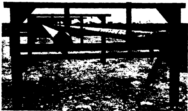
Figure 2-155. Station 2220 - Supports for Pipes
