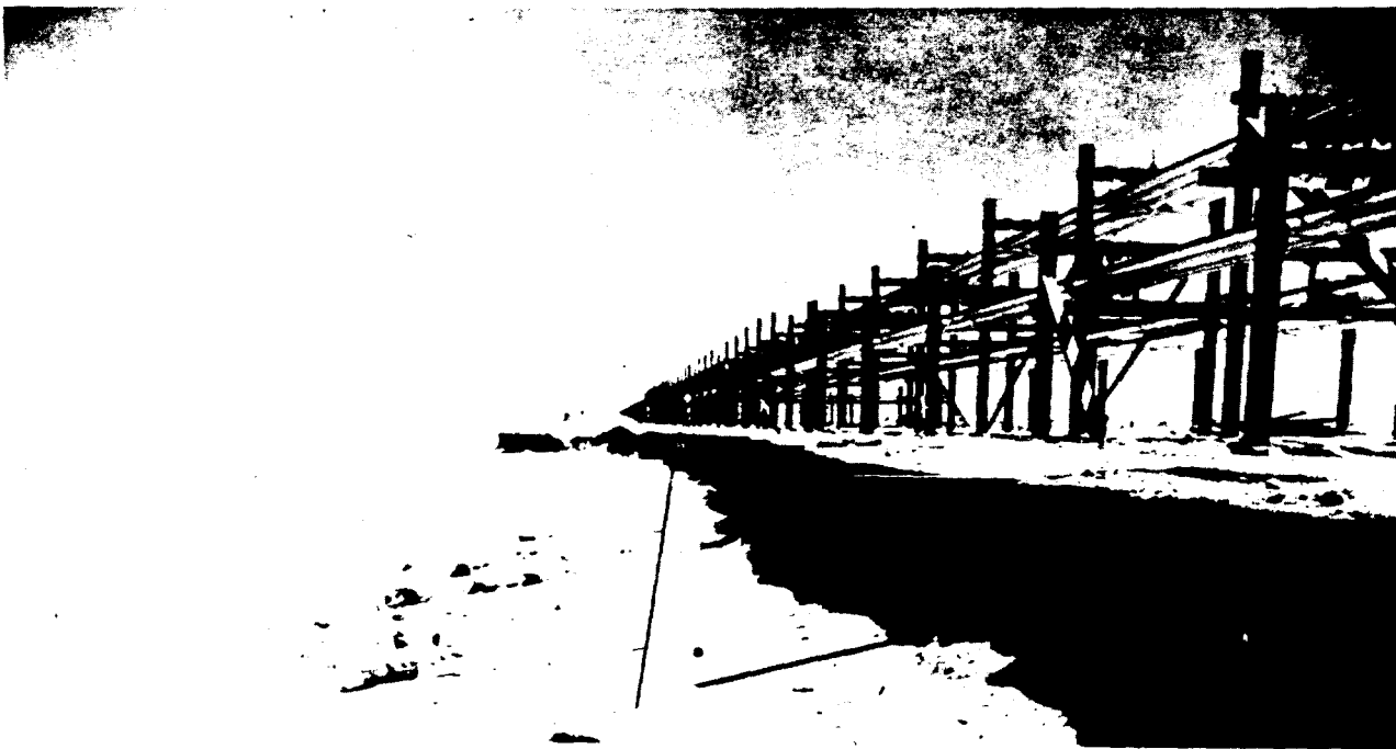
Figure 2-213. Charlie Causeway - Erosion from Wave Action
