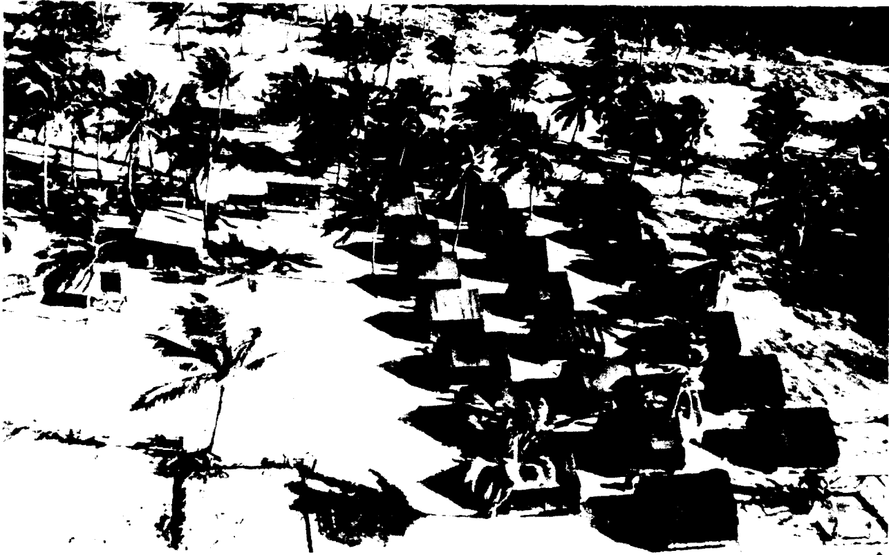
Figure 2-34. Temporary 50-Man Camp - Site Nan
