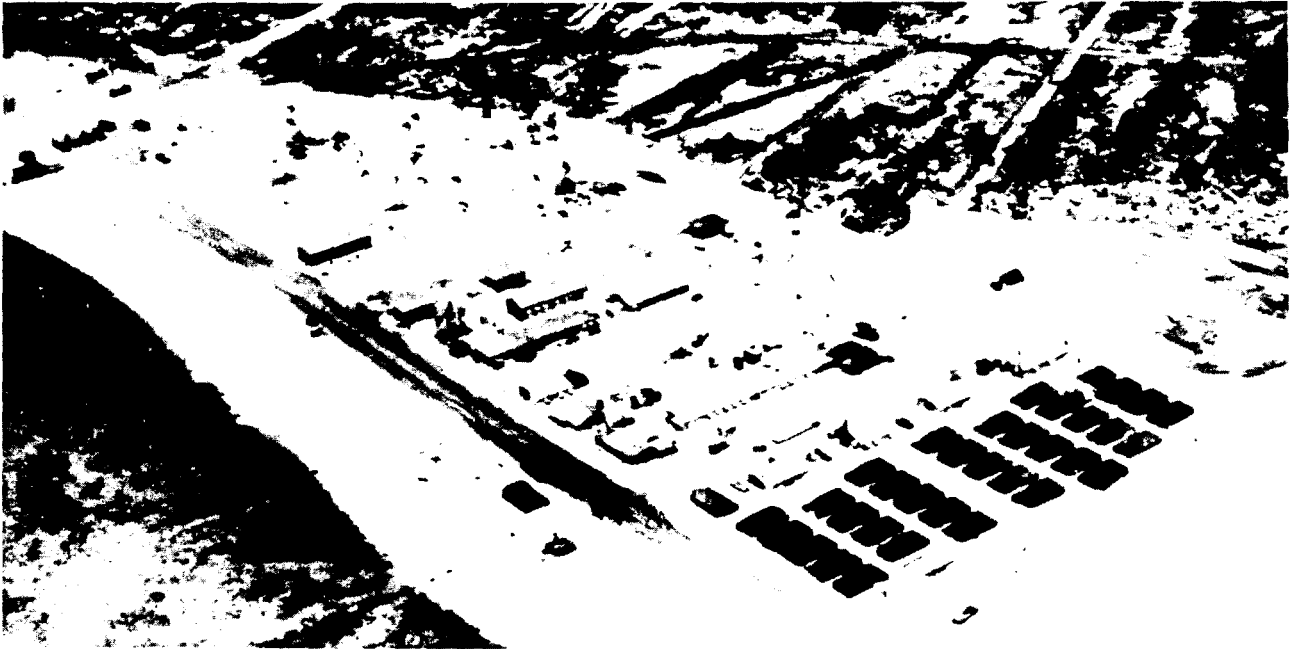
Figure 2-51. Aerial - Charlie Campsite Completed
