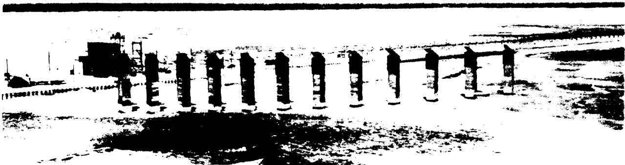
Figure 2-131. Station 1350 Series Completed
