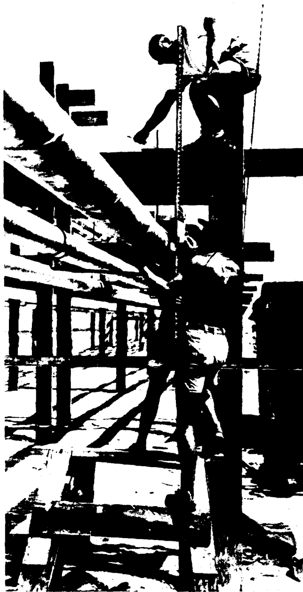
Figure 2-16. Vertical Alignment of Pipe Arrays
