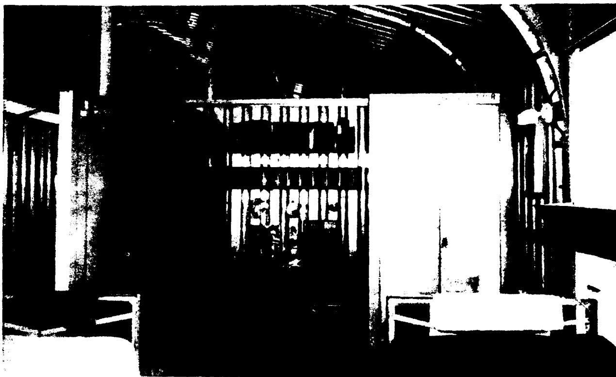
Figure 4-13. Barracks Room, Elmer Camp
