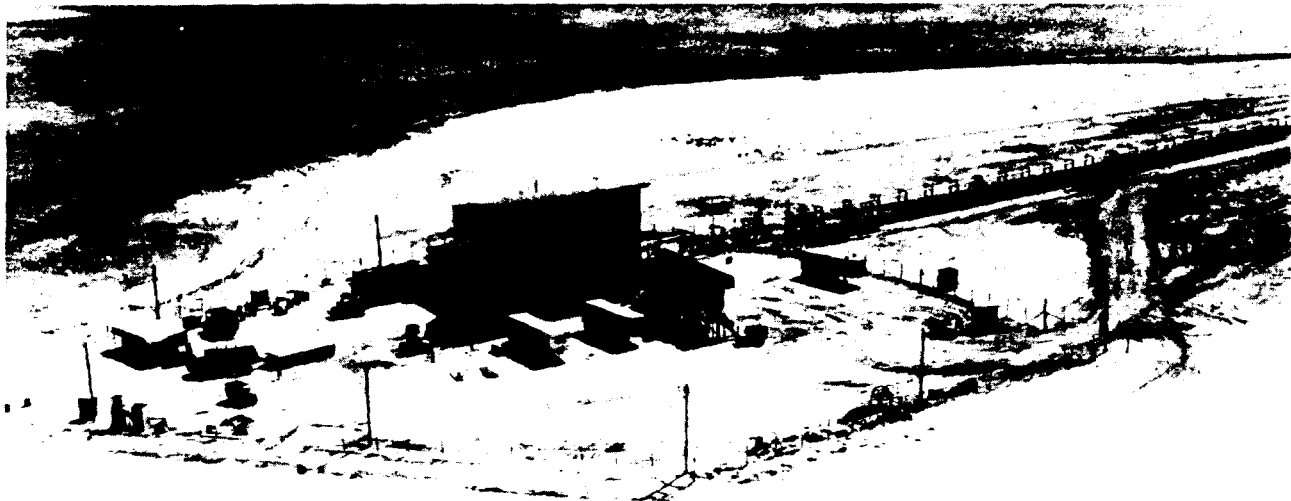
Figure 2-84. Station 60 Aerial View
