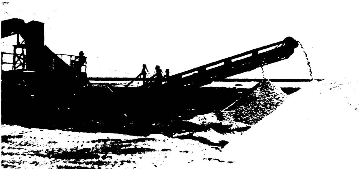
Figure 2-23. Crusher Plant at Site Charlie
