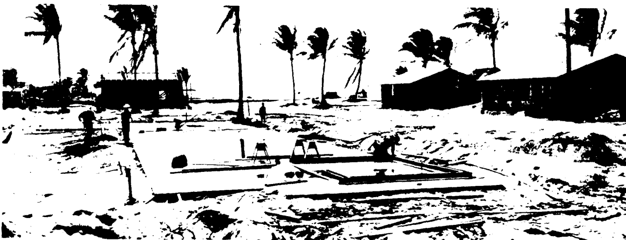
Figure 2-60. Pouring Mess Hall Slab - Fox Camp
