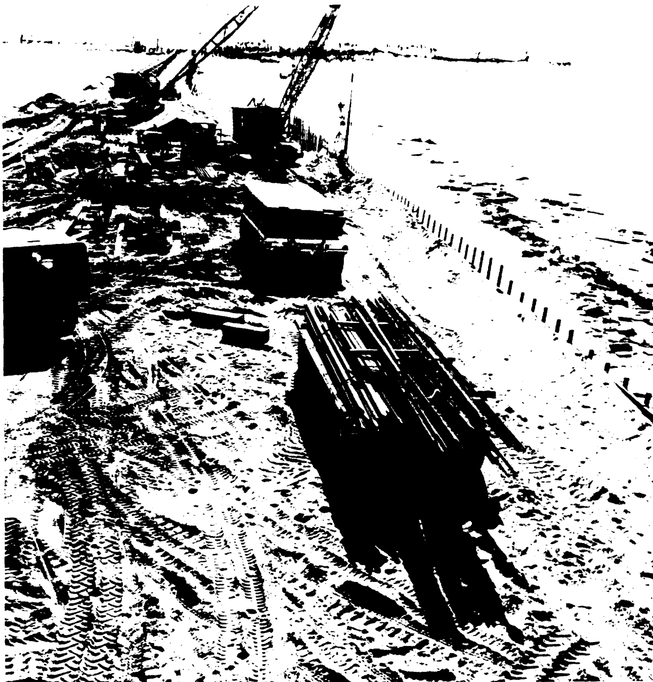
Figure 2-210. Charlie Causeway - Construction of Bulkhead
