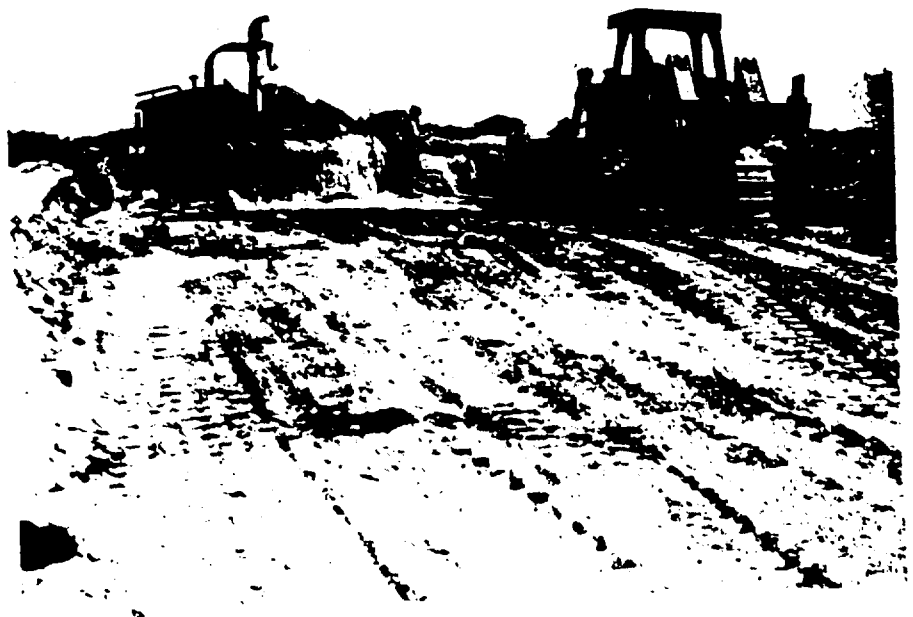
FIGURE 6-6. BACKBLADING OPERATION.
