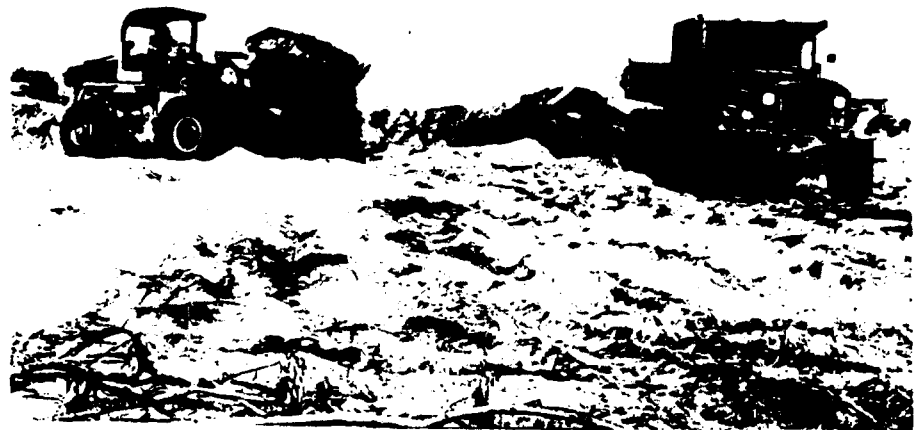
FIGURE 6-9. CONTAMINATED SOIL MOVEMENT.
