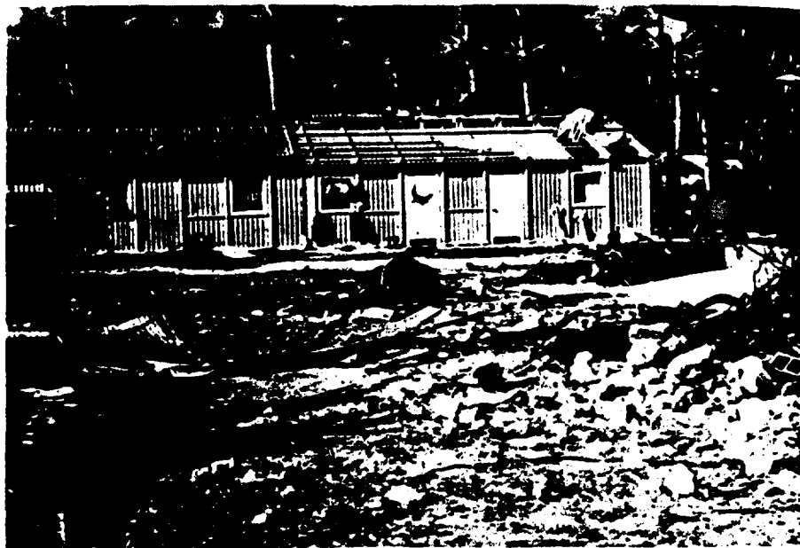
FIGURE 7-20. TYPHOON ALICE DAMAGE, BILLET.
