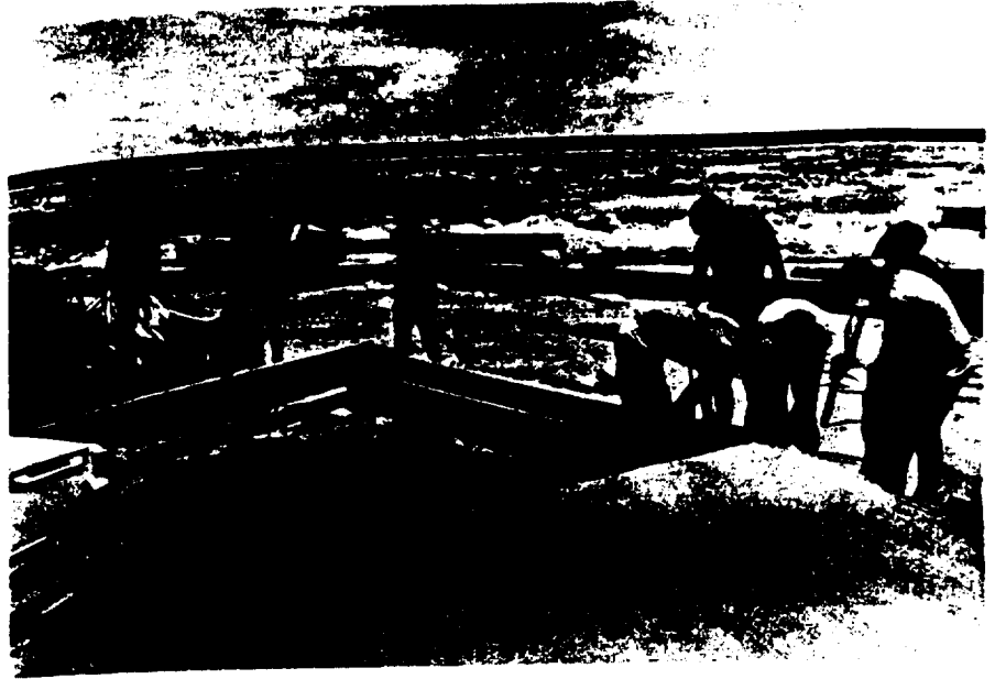
FIGURE 8-45. WOODEN CAP FORMS WITH TAPERED KEY.
