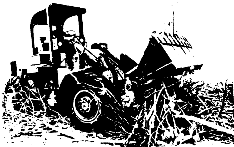
FIGURE 6-5. BRUSH REMOVAL USING FRONT LOADER.
