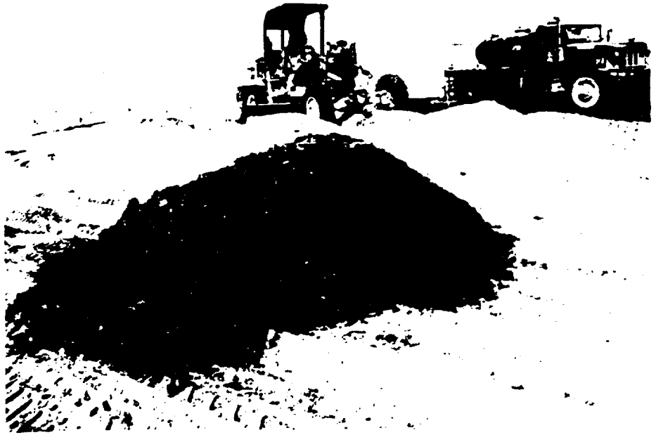
FIGURE 8-29. SPREADING SOIL WITH A GRADER.
