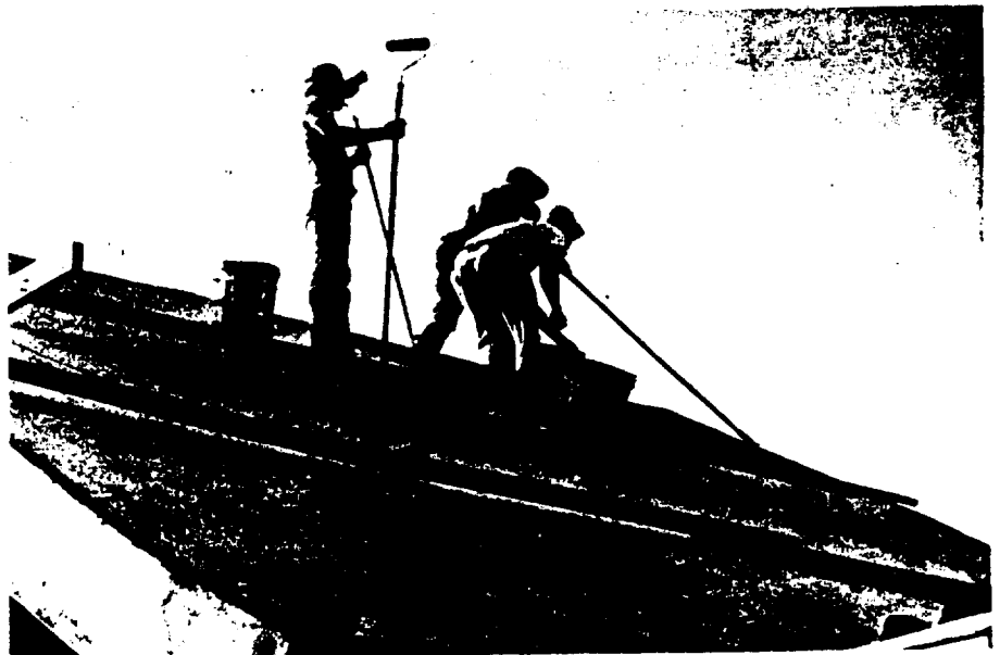
FIGURE 10-18. PAINTING THE ROOF.
