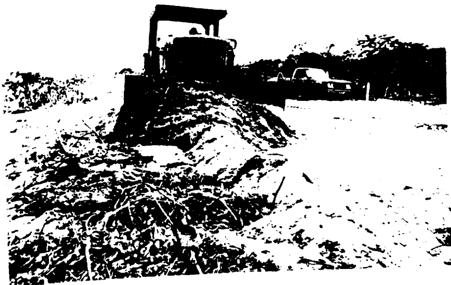
FIGURE 6-4. SOIL REMOVAL USING D8K DOZER.
