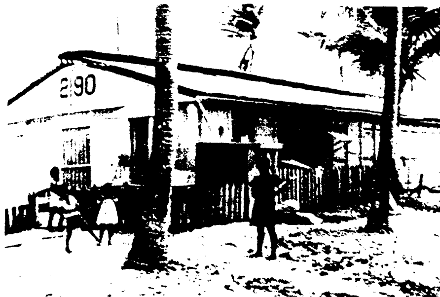
FIGURE 10-40. CONVERTED APARTMENT BUILDING ON JAPTAN ISLAND.
